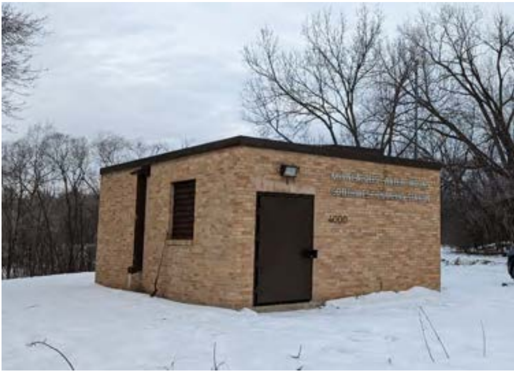
Photo of the existing SouthWest Pump Station.
