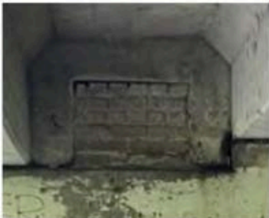
Filled utility blockout
