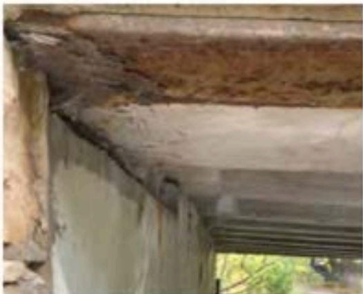
Steel lintel at north abutment
