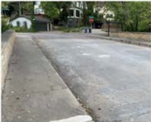
Deck Patching and joint repair
