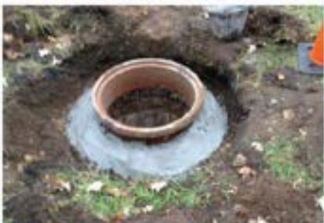
Infiltration & Inflow Repairs
