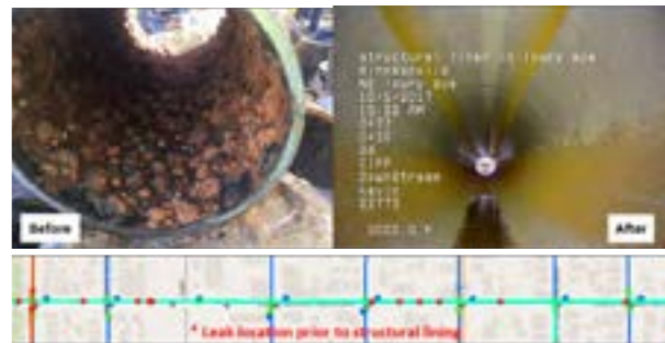
Water Main - Structural Lining
