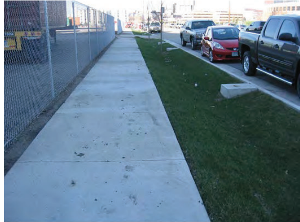
Vegetated Swale at 25 th Ave. SE
