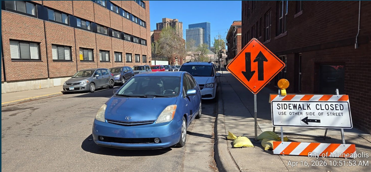
Centerpoint Traffic Control – Temp. 2-way from 18 th St. to Stevens
