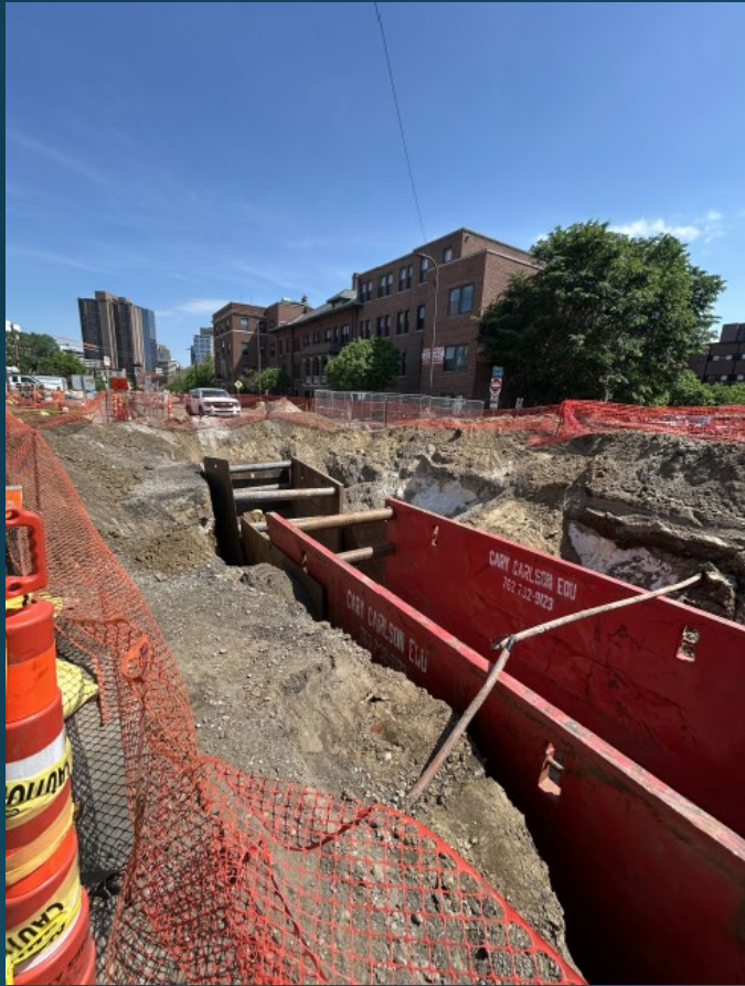
South of I-94 Bridge Activity (18 th St)
