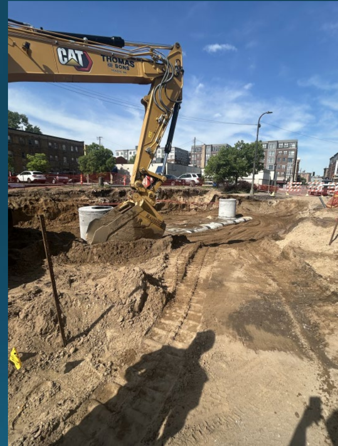
North of I-94 Bridge Activity (15 th St)
