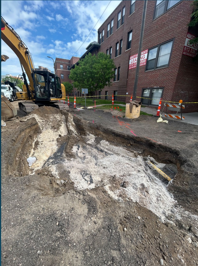
South of I-94 Bridge Activity (18 th St)
