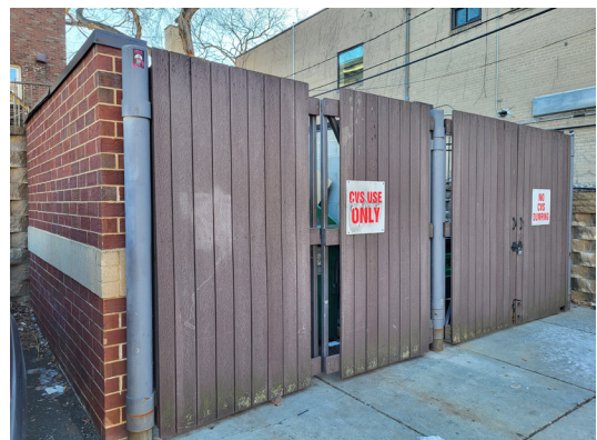
The trash enclosure at 15 Franklin Ave E is simple. It uses brick and wood pickets.
