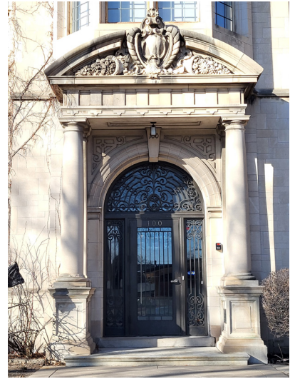
This stone entry at 100 22nd St E is a distinctive historic feature. The pediment above the door has carvings of fruits and flowers.
