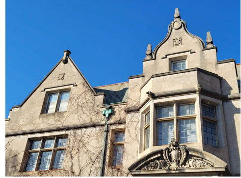
The house at 100 22nd St E has several historic roof features. The roof is covered with slate. The gutters are built into the roof. Stone parapets extend up from the roof. The one on the left is pointed. The one on the right is stepped and scalloped with carved finials.
