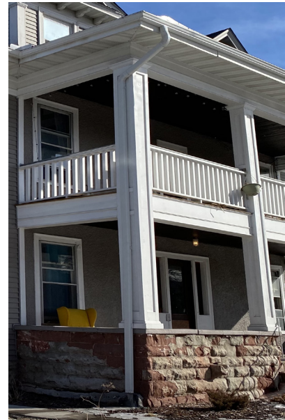
The square railing posts at 2511 1st Ave S are simple and do not mimic historic designs.
