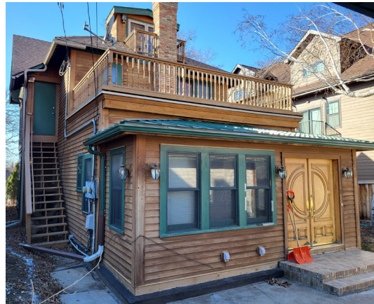
At 2417 1st Ave S, there is a one-story rear addition, built in 2003. It is smaller than the original building. The roof shape and material differ from the original building. The window pattern is contemporary and still compatible.
