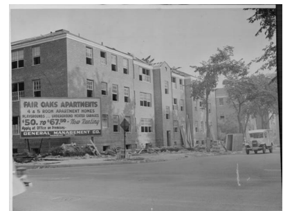
The Fair Oaks Apartments at 2421 3rd Ave S, built in 1939, were the last to be built during the period of significance. Courtesy of the Hennepin County Library James K. Hosmer Special Collections.
