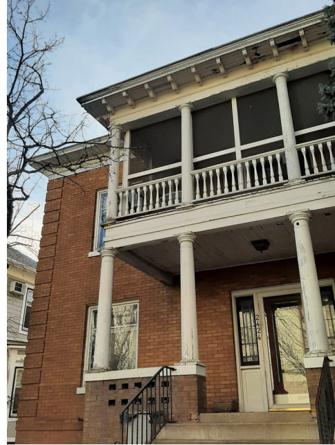
This two-story porch at 2424 Stevens Ave has historic architectural details that should be retained. Wood Tuscan columns support the structure. Turned wood railings line the second story.
